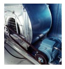
Figure 3 - Belt driven fan assembly
