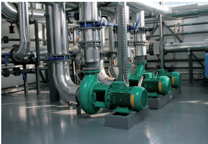
Figure 17: High potential savings with pump systems
